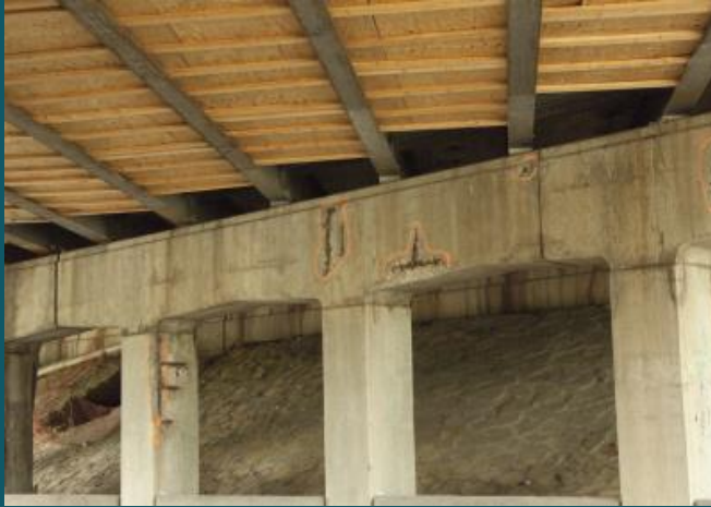
Plywood Under I-375 Bridge
